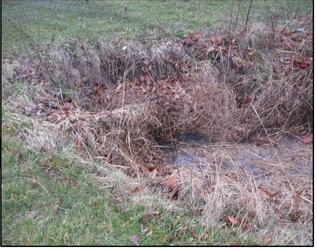
WEST SIDE SR 60 DITCH ALONG RES. #3503
