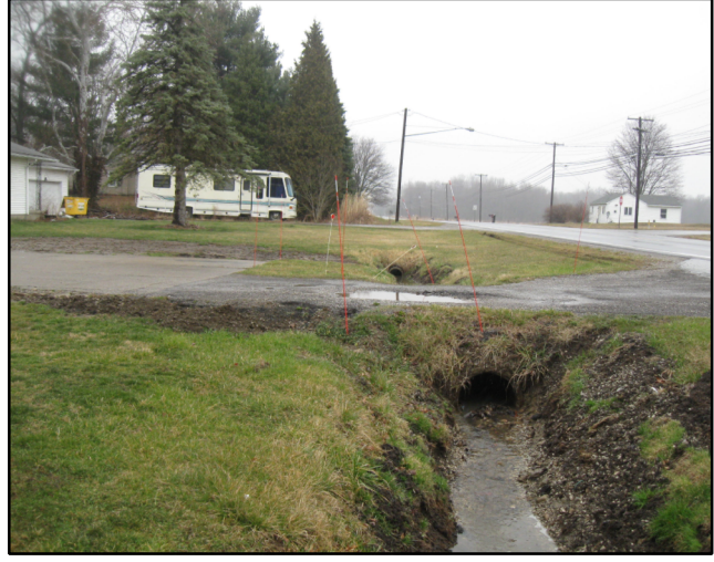
WEST SIDE SR 60 DITCH ALONG SR 60 NORTH
